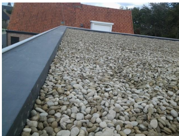
Foto dakplatform in EPDM ter illustratie
